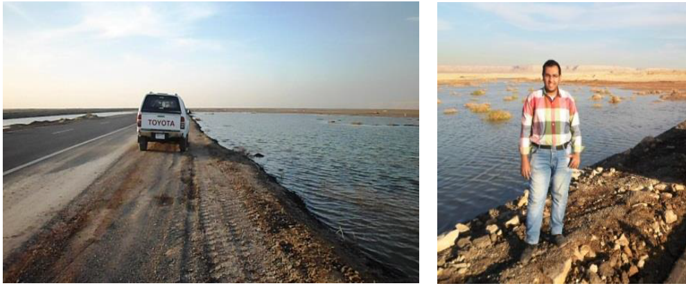
Fig (8): Field photographs showing the runoff water on both sides of El Sheikh Fadl – RasGharab road (20/11/2018).
